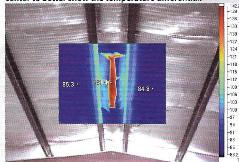
Thermal imaging picture of a roof line with Low-E™ Insulation. Note: The Low-E™ Insulation has been cut and pulled open in the center to better show the temperature differential.
